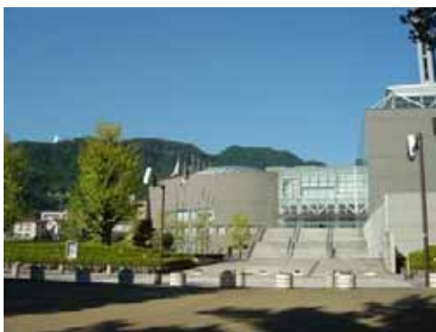
B-Con Plaza, Main Entrance
